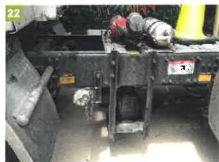
(21) A tanker dome clamp. (22) A PTO pump for filling aboveground tanks.
