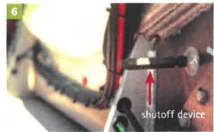
(6) An unmarked pneumatic breakaway emergency shutoff device (arrow) that is operated by the breaking off device.
